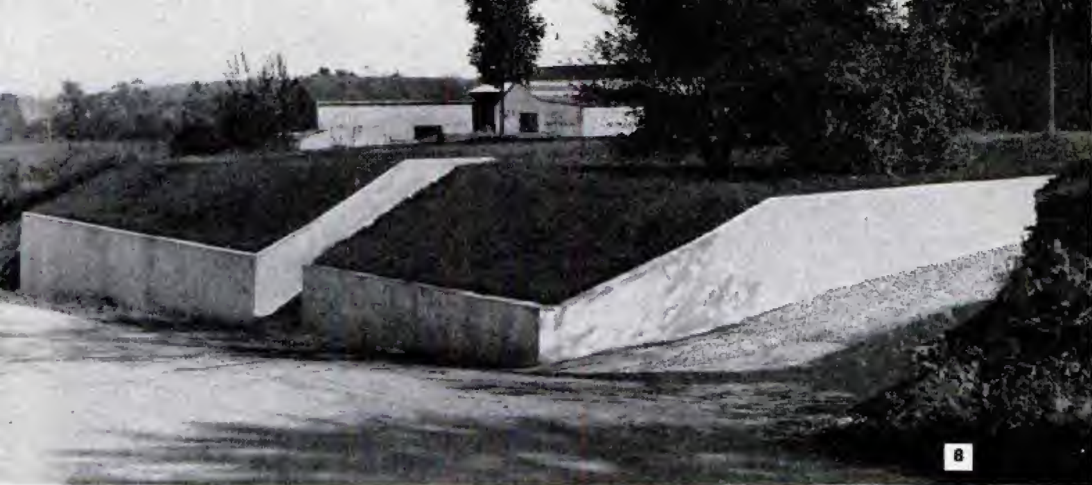
Photo courtesy Portland Cement Association
